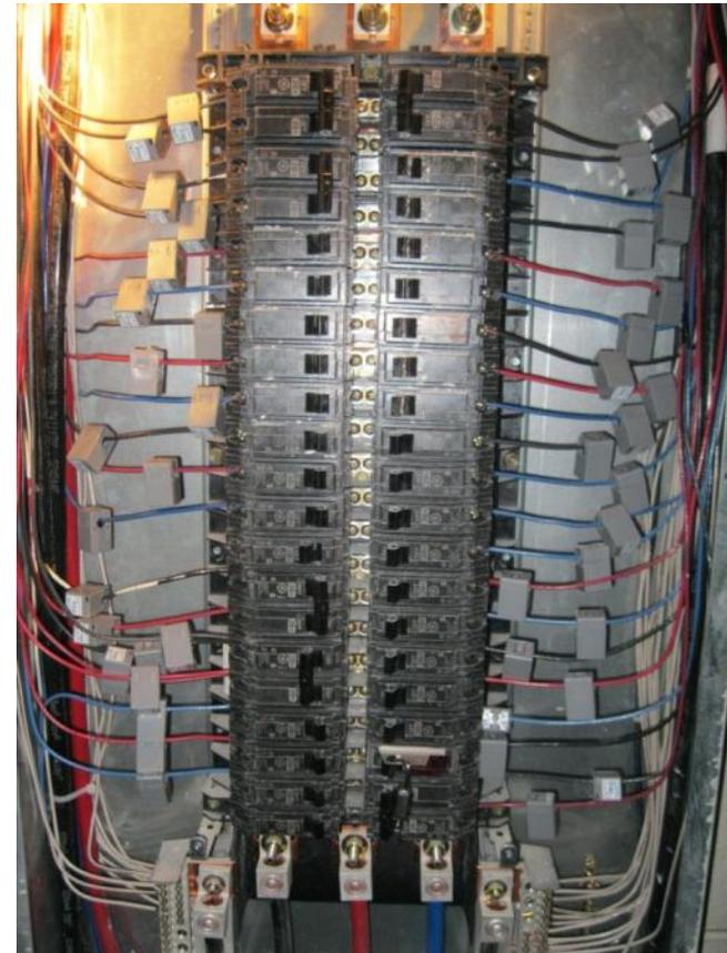
**Figure 74 Wireless current sensors installed in an electrical panel in Building 1219**
