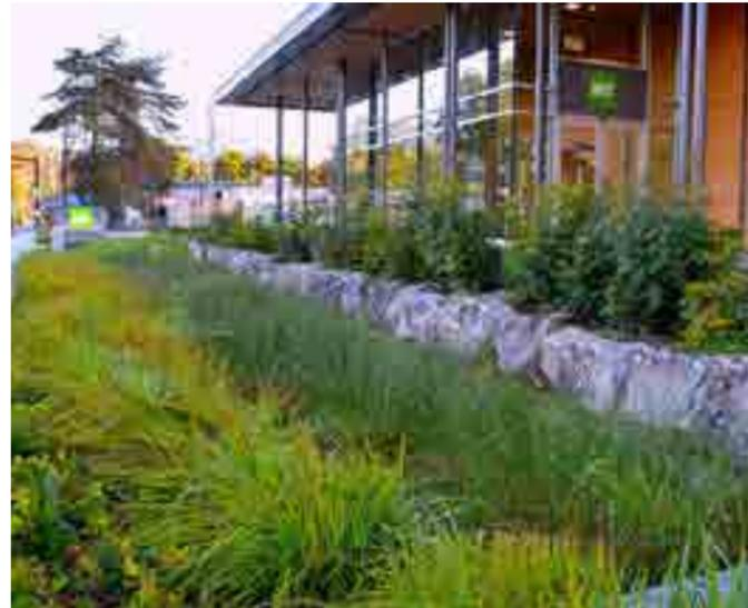
*Micro-bioretenction along building edges*
