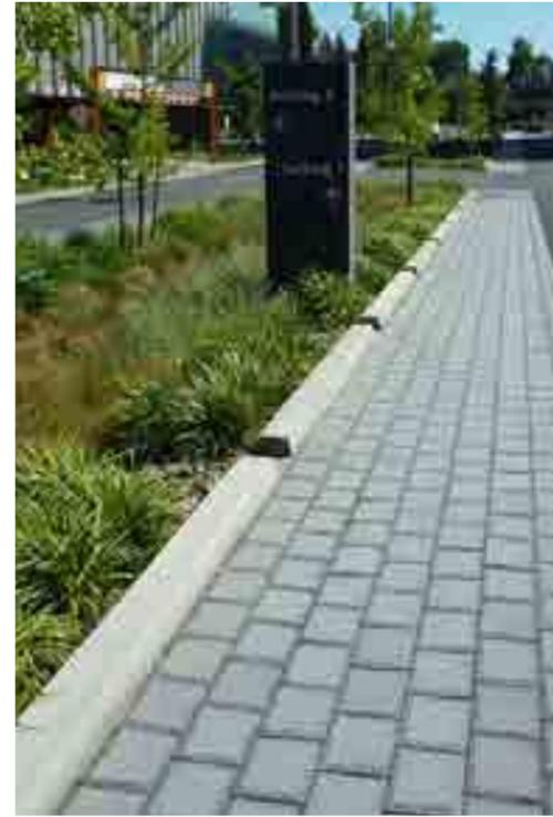
*Pervious paving with curb cuts*
