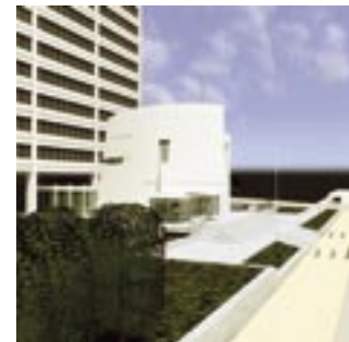
Entrance Pavilion, Richard B. Russell Federal Building, Atlanta, GA.
