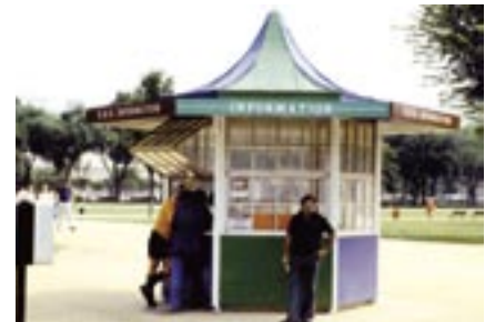
Freestanding kiosk with electrical service, National Mall, Washington, DC.
