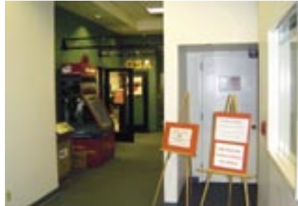
Ad-hoc signage such as these easels at the Phillip Burton Federal Building and U.S. Courthouse in San Francisco, CA may detract from a facility's image.
