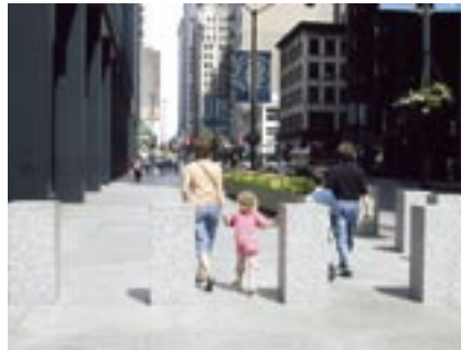
Bollards, Kluczynski Federal Building, Chicago, IL.
