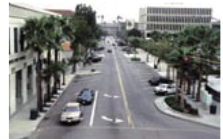
Traffic calmed downtown street with bulbout and angled parking, San Bernardino, CA.
