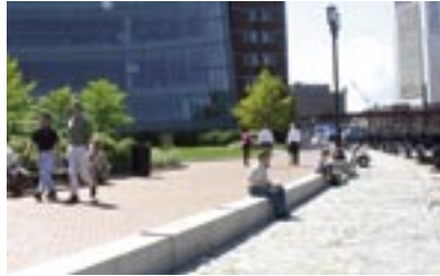
Security cameras are installed in the sidewalk light fixtures at the John Joseph Moakley U.S. Courthouse, Boston, MA.
