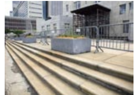
Security fencing and bulky planters create an unwelcoming atmosphere.
