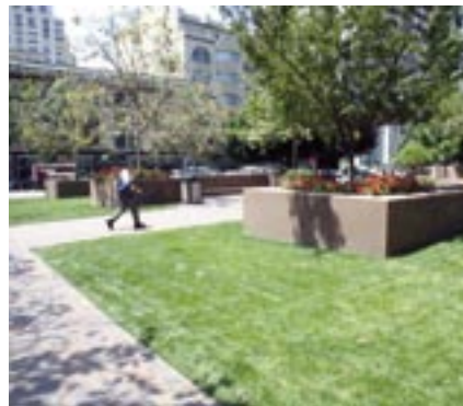
New lawn area, Edward J. Schwartz Federal Building and U.S. Courthouse, San Diego, CA.
