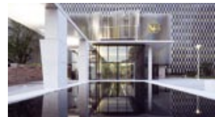
Richard Bolling Federal Building, Kansas City, MO, after renovation of interior and exterior public space.
