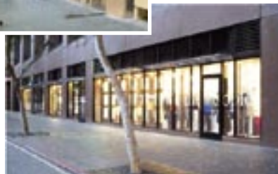
A false facade provides the appearance of a transparent ground floor at the Edward J. Schwartz Federal Building, San Diego, CA.
